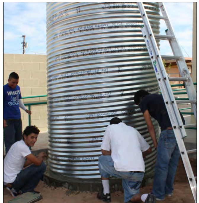
Students at YouthWorks, install a 2,100-gallon cistern through WMG's Schoolyard Water Education Program.
